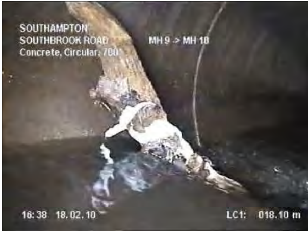
Photo: 117_7a, Tape No.: 1 18.1m, Obstruction, 40 % height/diameter loss, Remark: TREE TRUNK
