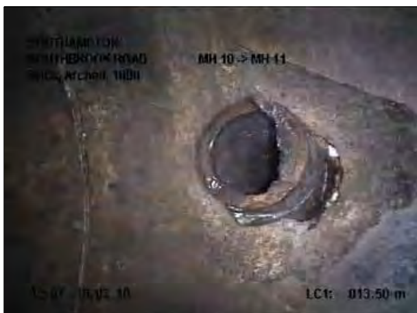
Photo: 11_16a, Tape No.: 1 13.5m, Connection, at 12 o'clock, dia 100 mm, intrusion 150 mm
