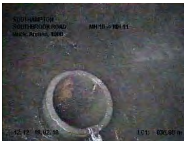
Photo: 146_22a, Tape No.: 1 36.8m, Connection, at 09 o'clock, dia 150 mm, intrusion 80 mm
