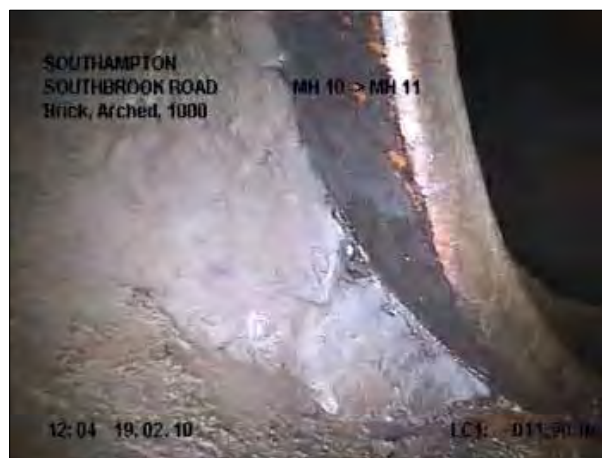
Photo: 11_15a, Tape No.: 1 11.9m, Connection, at 09 o'clock, dia 350 mm, intrusion 50 mm
