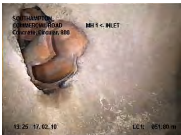
Photo: 24_21a, Tape No.: 1 51.8m, Connection defective, at 09 o'clock, dia 150 mm, intrusion 150 mm
