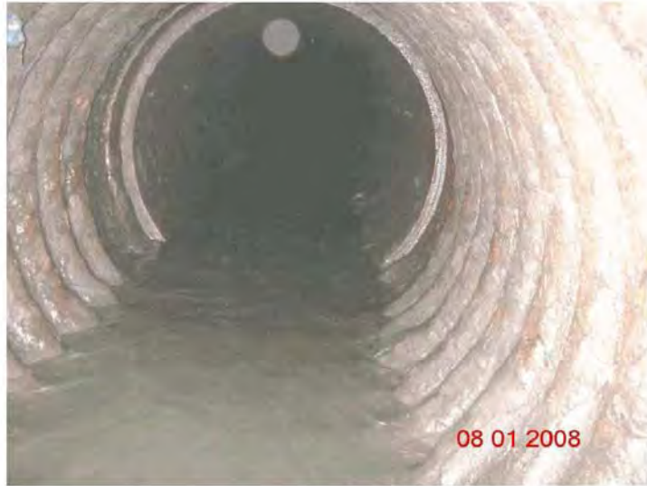
Photograph No 7 Corrugated Steel Section
