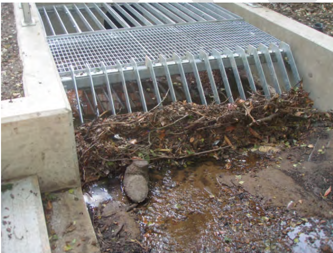
Figure 8. Recently constructed trash screen at upstream section of culverted section.
