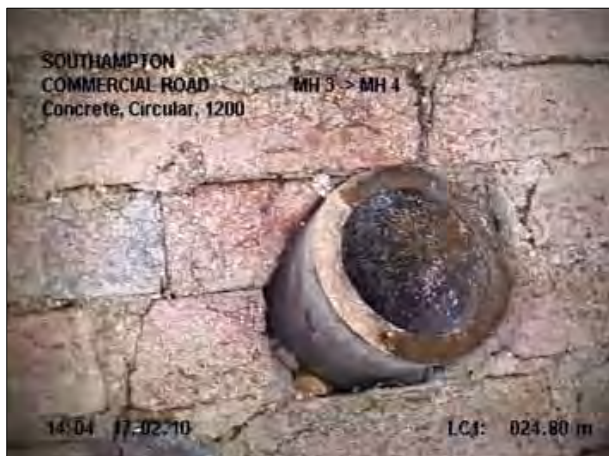
Photo: 51_11a, Tape No.: 1 24.8m, Connection, at 11 o'clock, dia 150 mm, intrusion 100 mm
