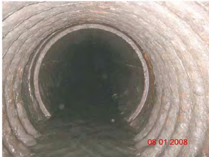
Photograph No 8 Corrugated Steel Section
