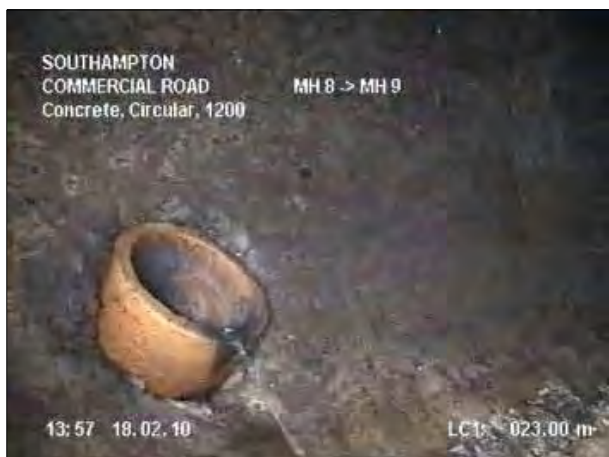
Photo: 106_7a, Tape No.: 1 23m, Connection, at 10 o'clock, dia 150 mm, intrusion 100 mm
