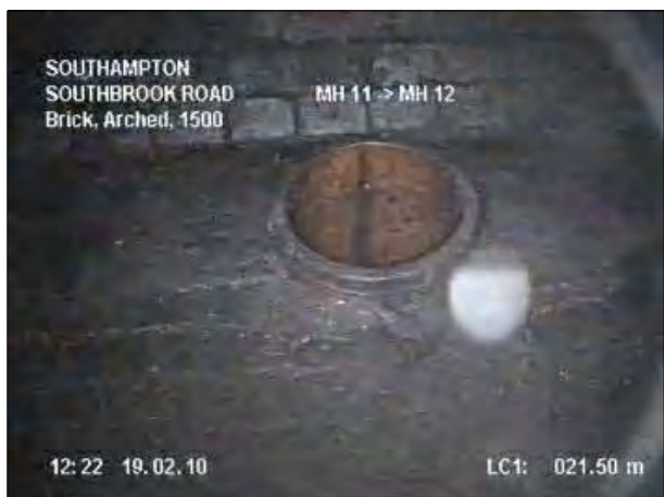
Photo: 157_6a, Tape No.: 1 21.5m, Connection, at 11 o'clock, dia 200 mm, intrusion 20 mm
