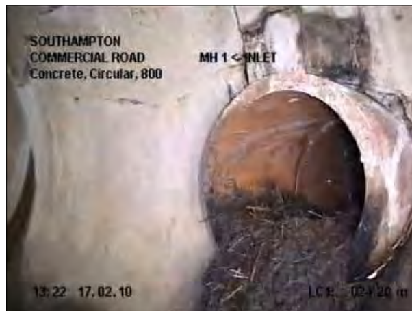
Photo: 17_15a, Tape No.: 1 24.2m, Connection, at 02 o'clock, dia 225 mm, intrusion 100 mm
