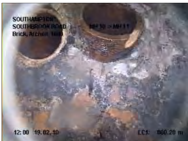
Photo: 128_6a, Tape No.: 1 0.2m, Connection, at 01 o'clock, dia 150 mm, intrusion 100 mm
