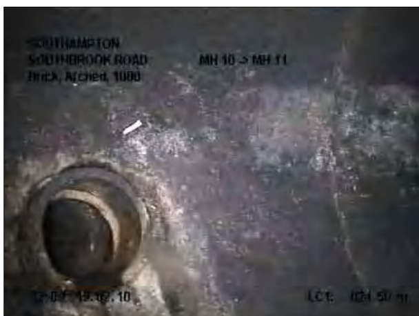
Photo: 11_18a, Tape No.: 1 24.5m, Connection, at 12 o'clock, dia 100 mm, intrusion 40 mm
