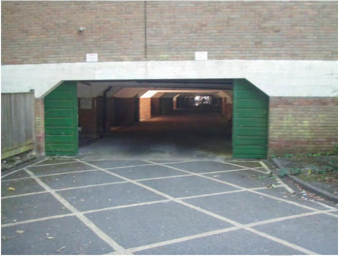
Figure 6. Garages situated under Grenville Court prevent fluvial flooding to properties above.
