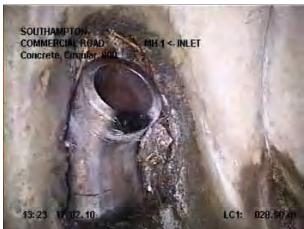
Photo: 18_16a, Tape No.: 1 28.9m, Connection, at 09 o'clock, dia 150 mm, intrusion 40 mm
