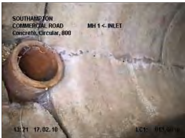
Photo: 14_12a, Tape No.: 1 13m, Connection, at 10 o'clock, dia 150 mm, intrusion 80 mm
