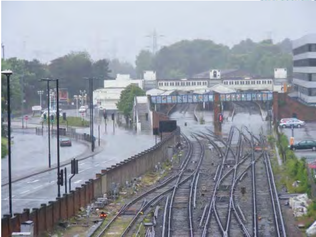
Figure 3: Central Station & Western Esplanade
