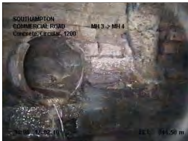
Photo: 53_13a, Tape No.: 1 44.5m, Connection, at 08 o'clock, dia 225 mm, intrusion 80 mm
